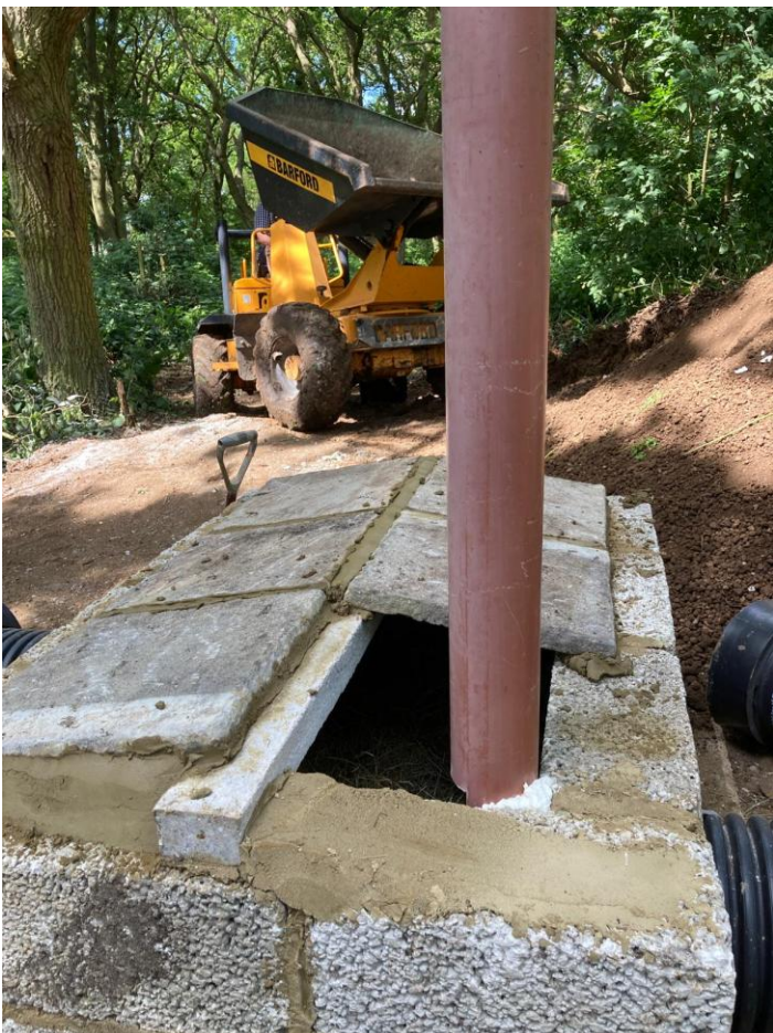
5. Lintels are concreted into place across the middle of the chamber and paving slabs are laid over the top on both sides.
